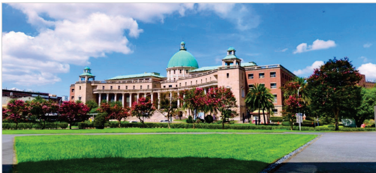
FIGURE 4 Front view of Administration Building at Asia University.
